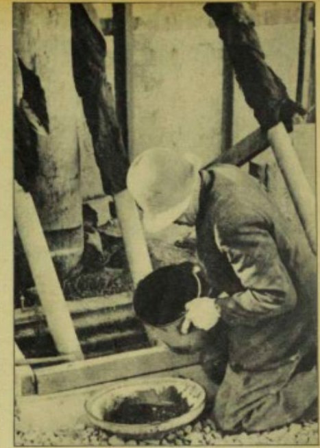
Collecting Mercury Gas from retorts passes through pipes wrapped with wet sacking. Pipe ends are just covered by water. When mercury forms, it sinks to bottom in buckets.
