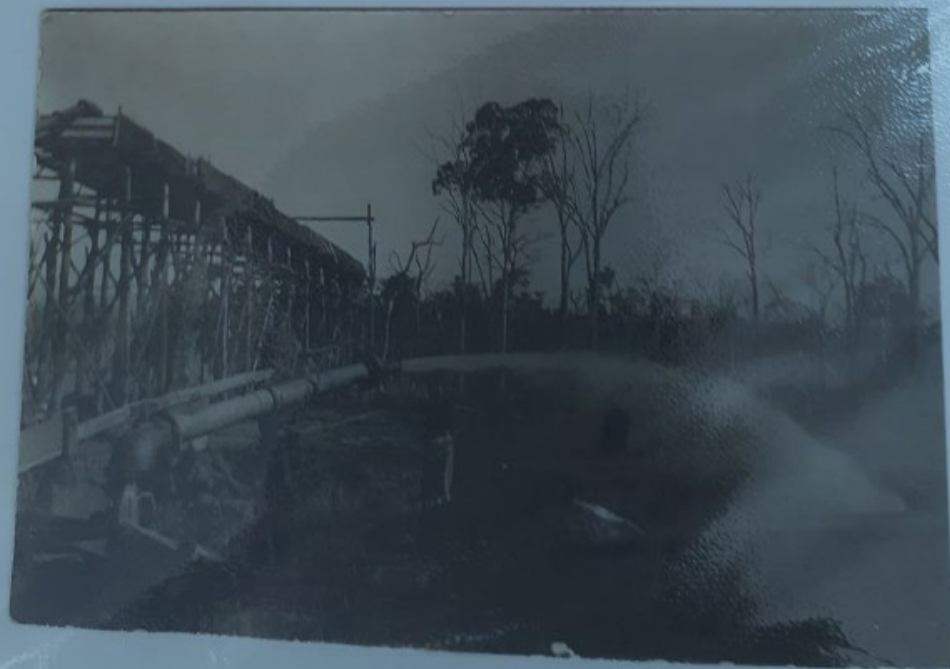
27. "QUICKSILVER PLANT IN OPERATION 23.3.33 SLUICE BOXES SHOWING SLURRY POURING OUT OF THE TAIL END AFTER SAVING QUICKSILVER. A.W. WILSON, (D & H WILSON) KILKIVAN."
