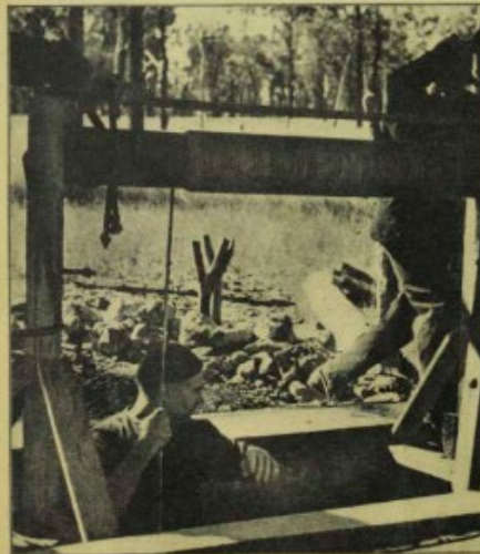
Man-Power Several shafts have been sunk at Cinnabar. Cost of recovering ore is relatively small, as little equipment is needed. Miners descend by windlass, scull ore in bucket aloft by same method.
