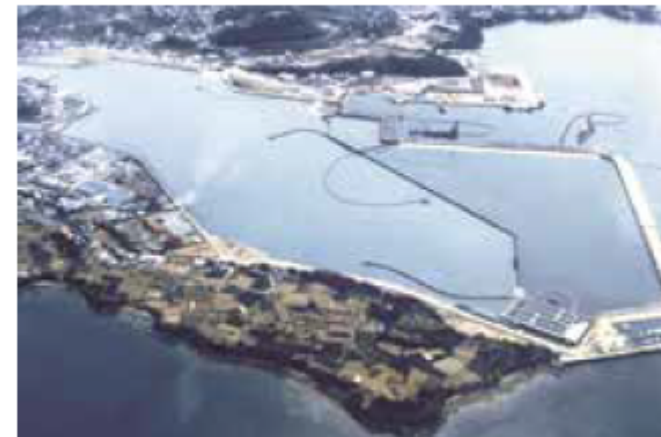
Dredging using a Cutterless Pump Dredging Ship
