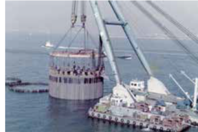
Construction of the Reinforced Shore using Steel Sheet Pile Cells
