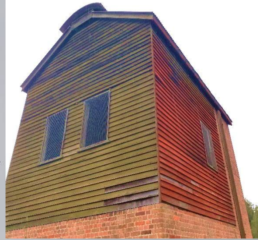
Retort House SW corner
