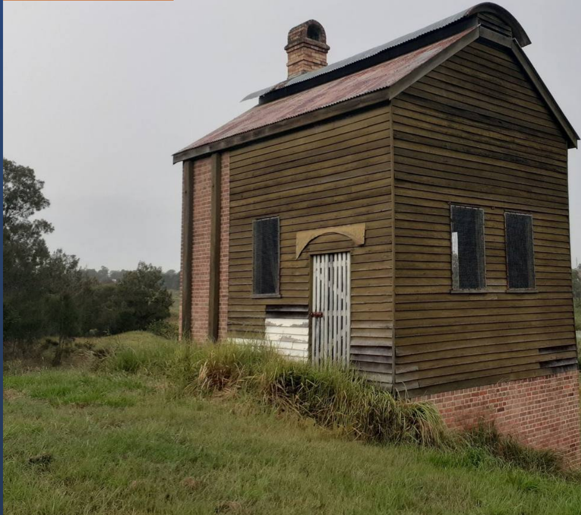
Retort House 29 March 2023 NW corner
